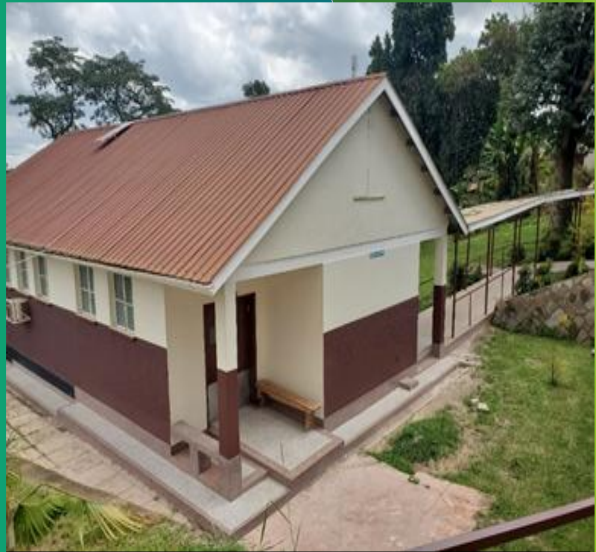
Theater rehabilitation at Buwambo HC IV
