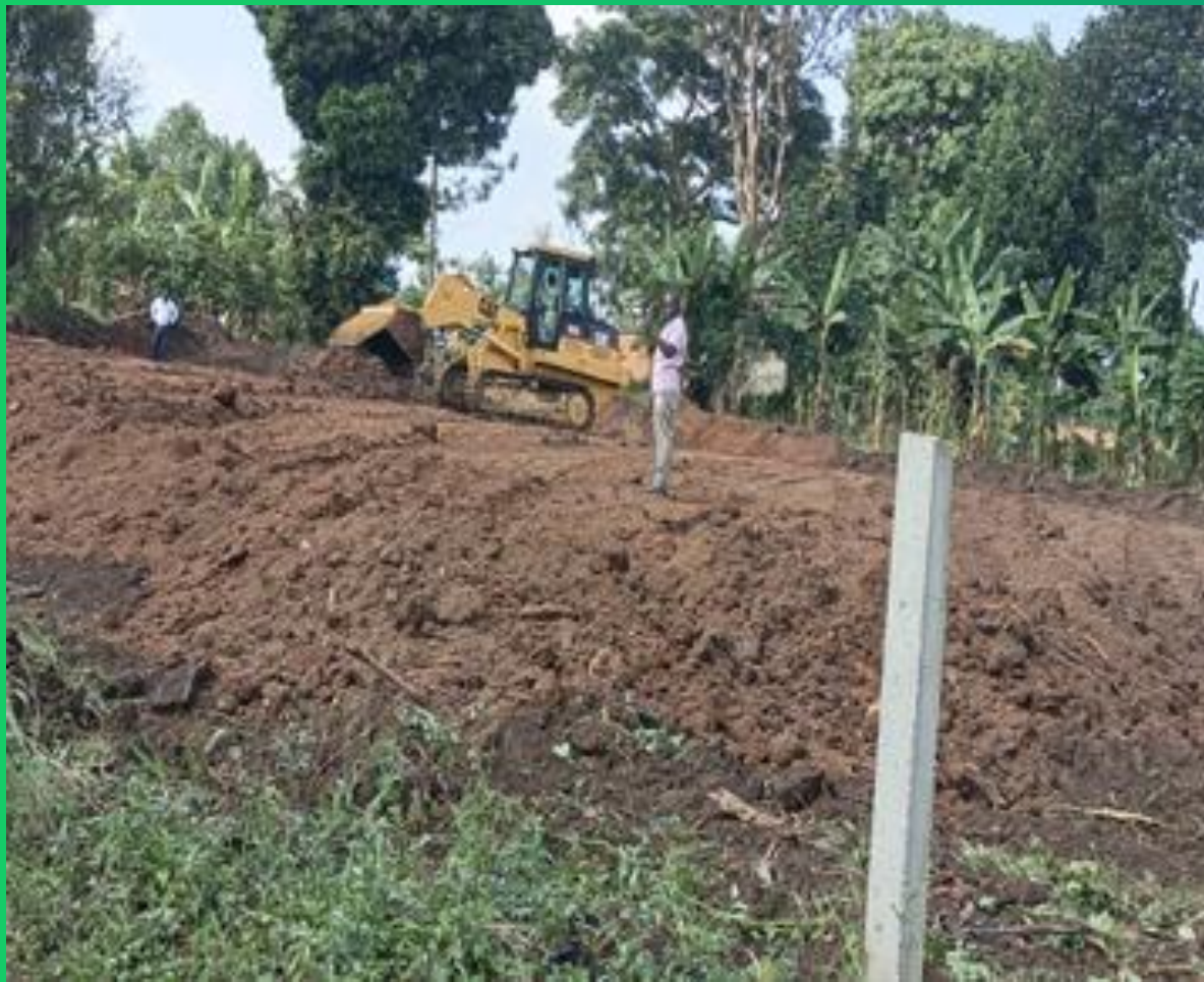
Site clearance for construction of staff Quarters at Ttikalu HC III completed under MoDVA Engineering Brigade
