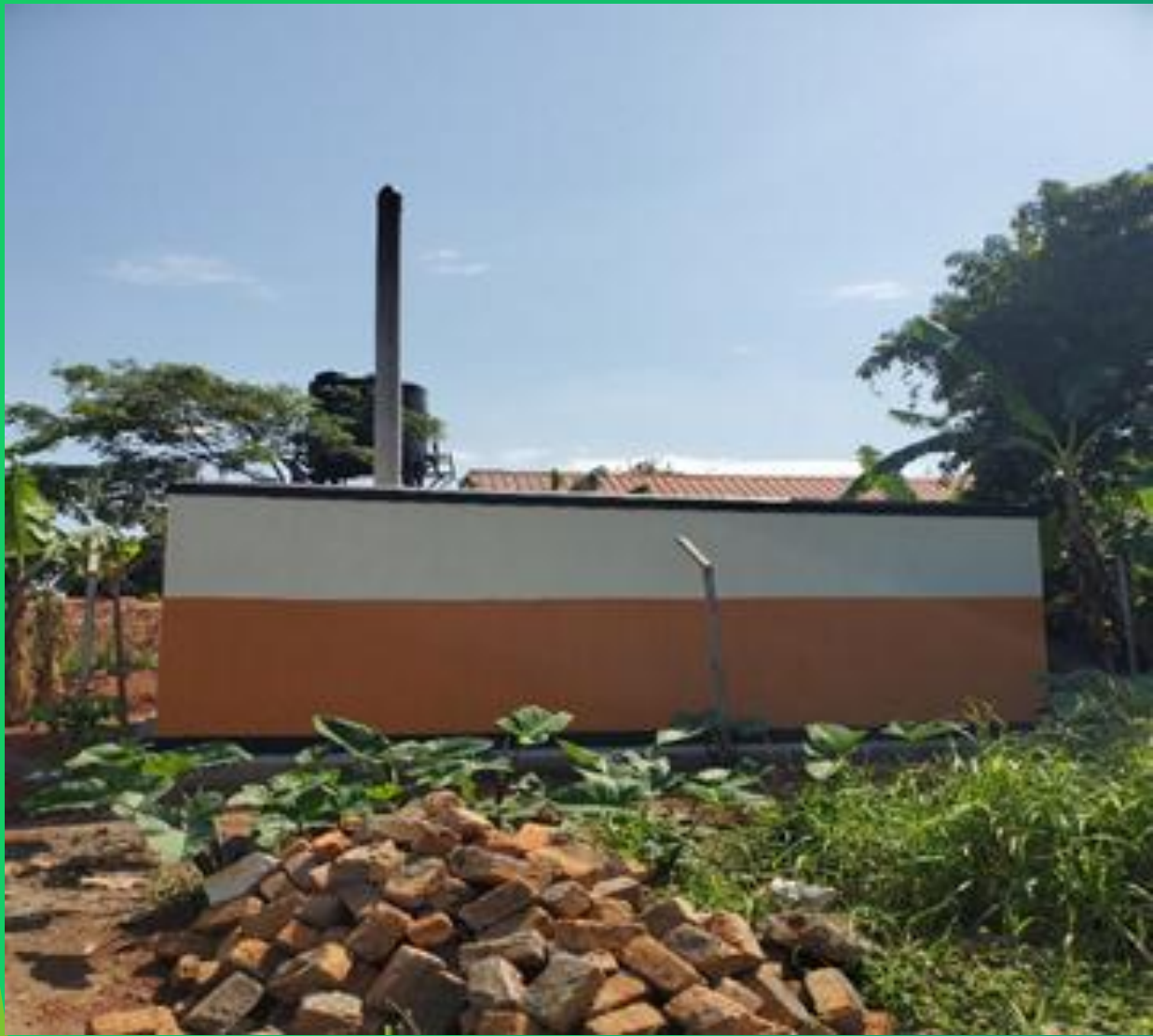
Construction of placenta pits for Næssolo Wamala and Nabweru HC III
